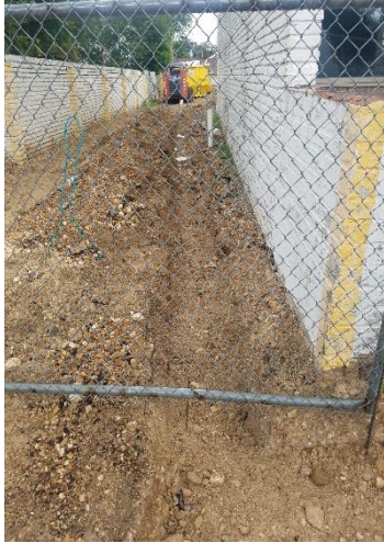
Trench for water line to Building 2
