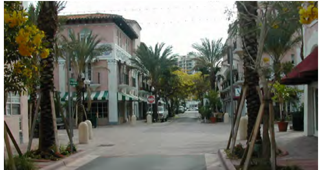
An example of a curbless intersection that features bollards and a high degree of spatial enclosure, resulting in slow driving speeds.
